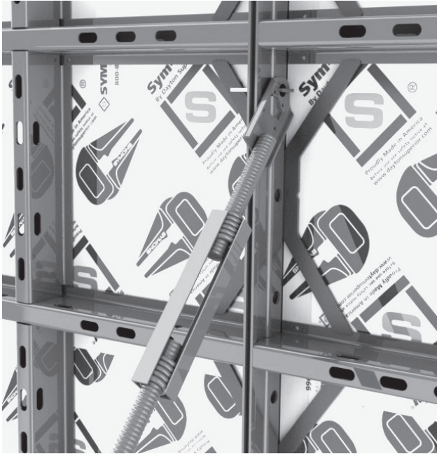
Turnbuckle to Siderail
