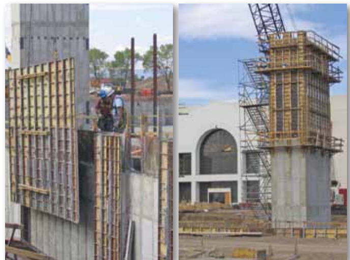
Gates Gang Form Adapters are available in : 4', 6', 8', 10', and 12' lengths and easily spliced together
